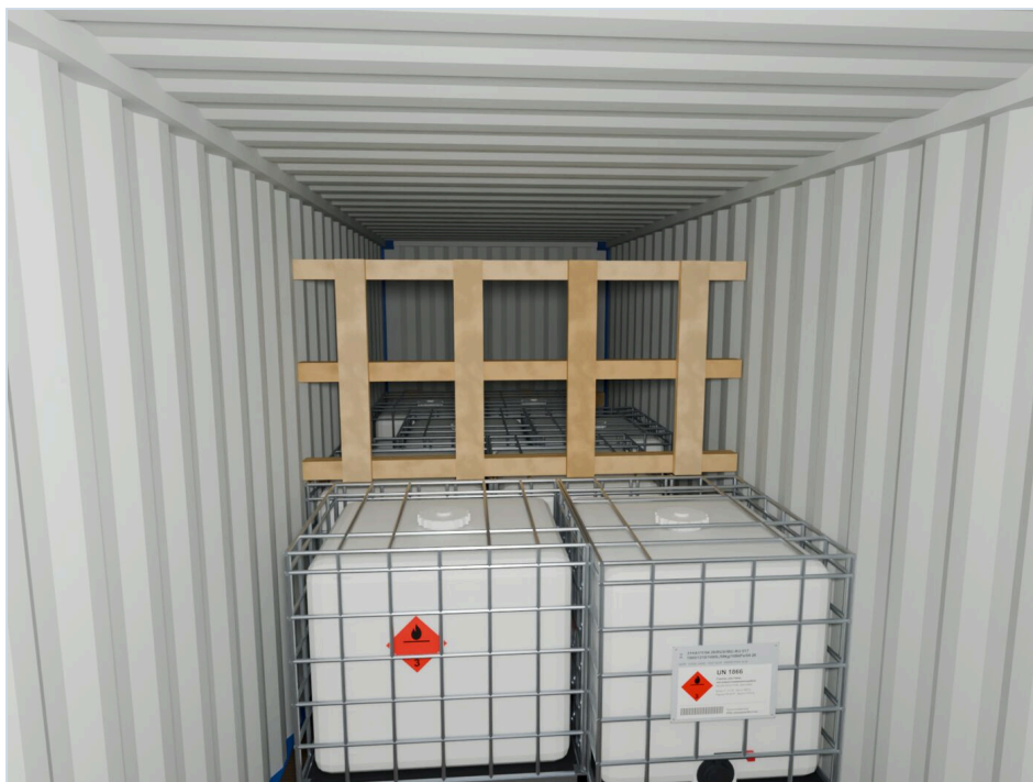
STAGE PHOTO 09 Second-tier shield on the end-wall side: 3 bars pos. 6, 4 posts pos. 10
